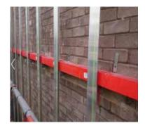
Teflon coated fixings and washers were used on the systems components to reduce friction and provide isolation between dissimilar materials.
