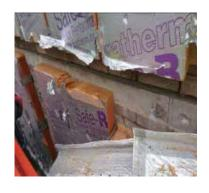
Work commenced by removing Reynabond pannels from the gable end of Salix Court. Once the task had been completed the operatives then began to remove each T rail from the carrier system along with insulation and fire break to expose the buildings brick work. Any historic penetrations in the brick substrate were then injected with EPDM sealant to protect the structure from water and air ingress.
