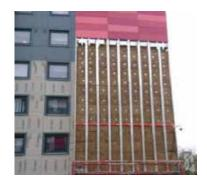
Once installation of the Fire break had been completed operatives then began installing 110mm Knauf Earthwool Dritherm Cavity Slab to the brick substrate. The insulation was then directly fixed to the building using 6 number plastic tie back fixings with spreader washer and 2 number stainless steel fire rated insulation fixings.
