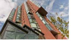
The splayed sandstone cladding and curtain-walled shards provide the majority of the apartments with a southerly view on this multi-cantilevered scheme.
