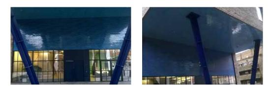
Fastclad Brick Slip Rainscreen was used on the tower elements of the main block, the balconies as well as the first and second floors of the main building for its weight, ease of installation and its fire properties. Pearl blue glazed brick slip was used a eye catching feature on the façade, expertly colour matched and mortared.
